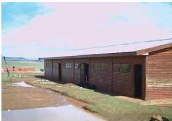
1.3.6.8. Wood used as building material for walls on site
