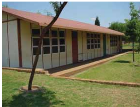
1.3.6.8. Wood used as building material for walls on site
