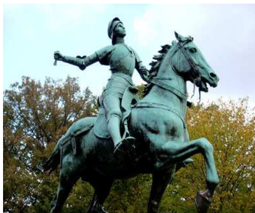
Can you see the green coating forming on this copper statue?
