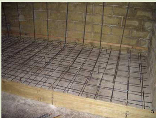
A piece of floor being prepared.
