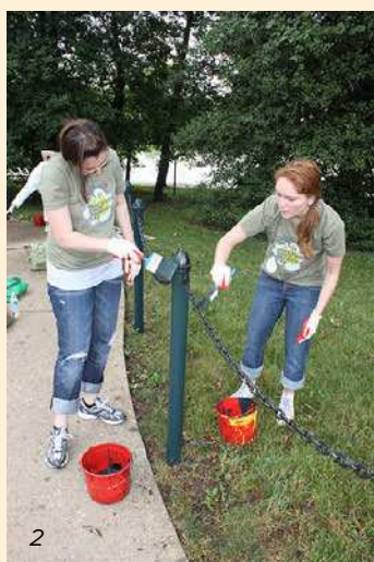
These people are painting the iron poles and fences.
