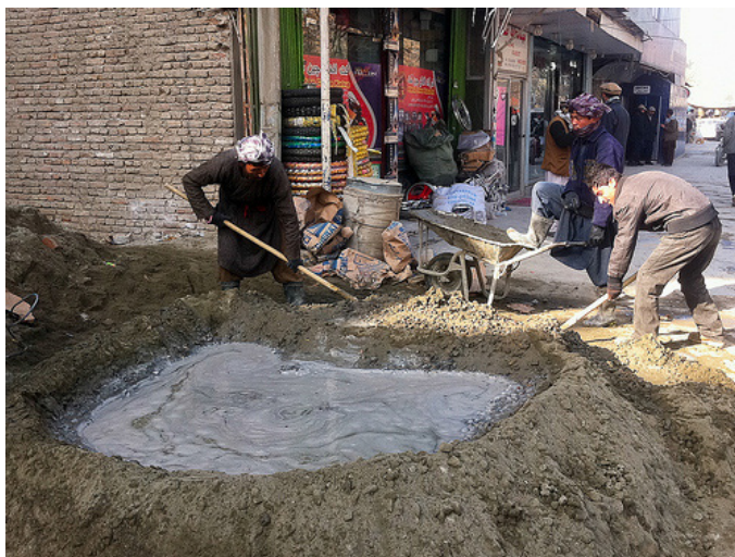
Mixing cement using spades.
