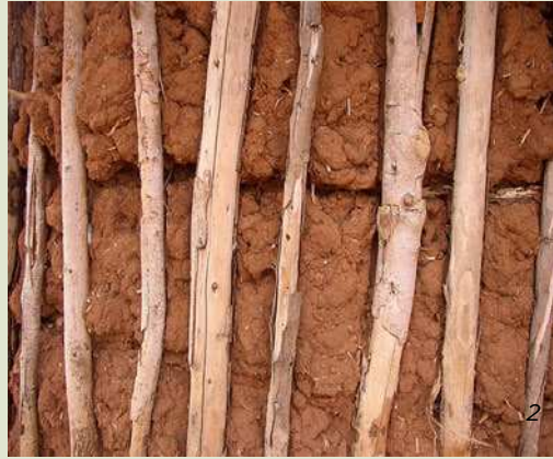
The wall of a mud house with a stick frame.
