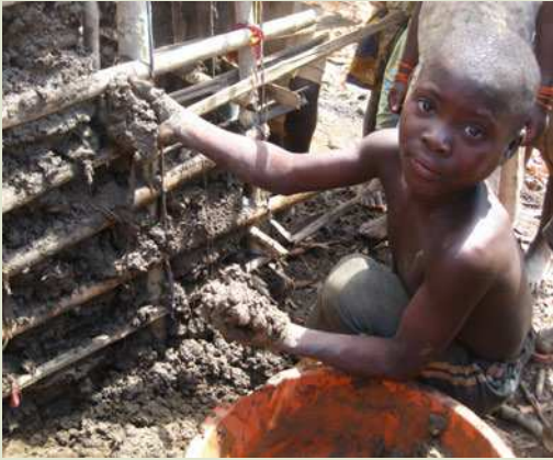
A boy helping to build a mud wall.
