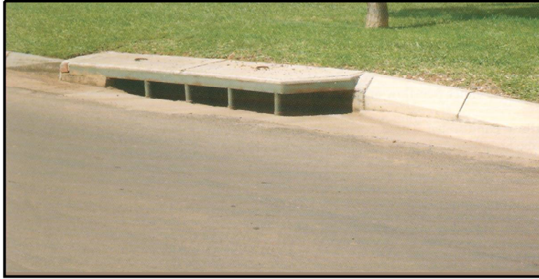
Figure 4.7: Kerb Inlet
